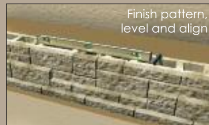
Compact on block and behind
