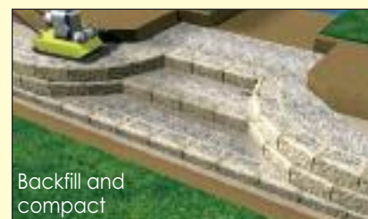
Install wall out from stairs
