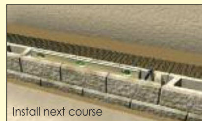
Install AB Reinforcement Grid
